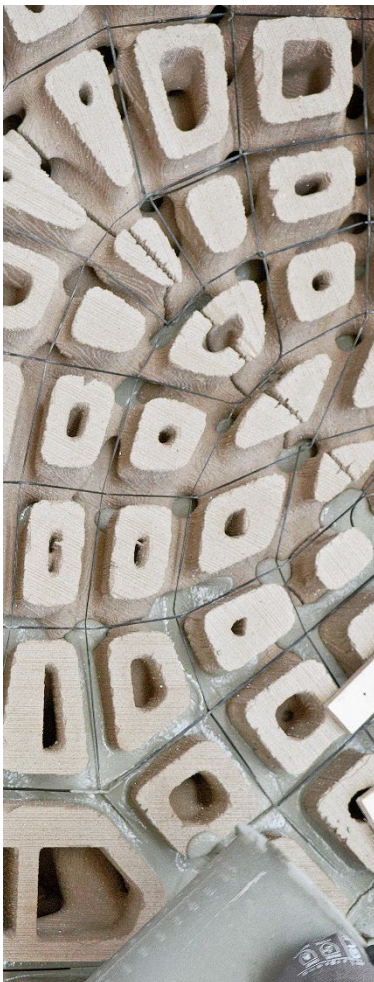
Casting of filigree fiber-reinforced concrete structure into sand formwork
